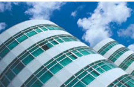
SentryGlas® Installation: Hospital, Florida
