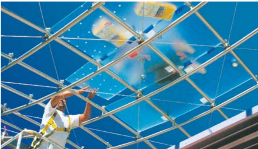
SentryGlas® Installation: Overhead Glazing
