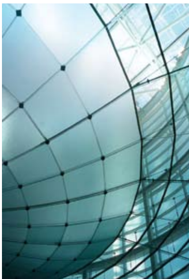
SentryGlas® Installation: Courthouse, Arizona
